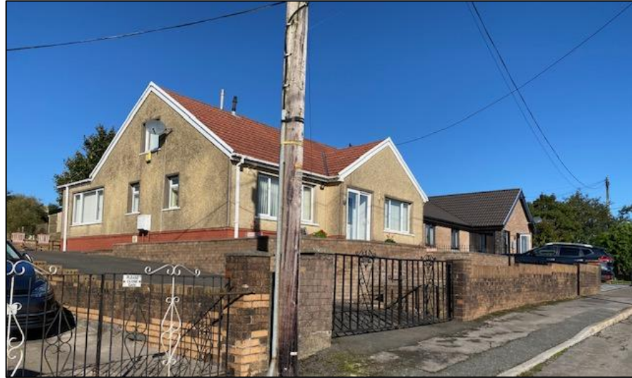
Photograph 8 – Typical Bungalows Established at Western Crescent
