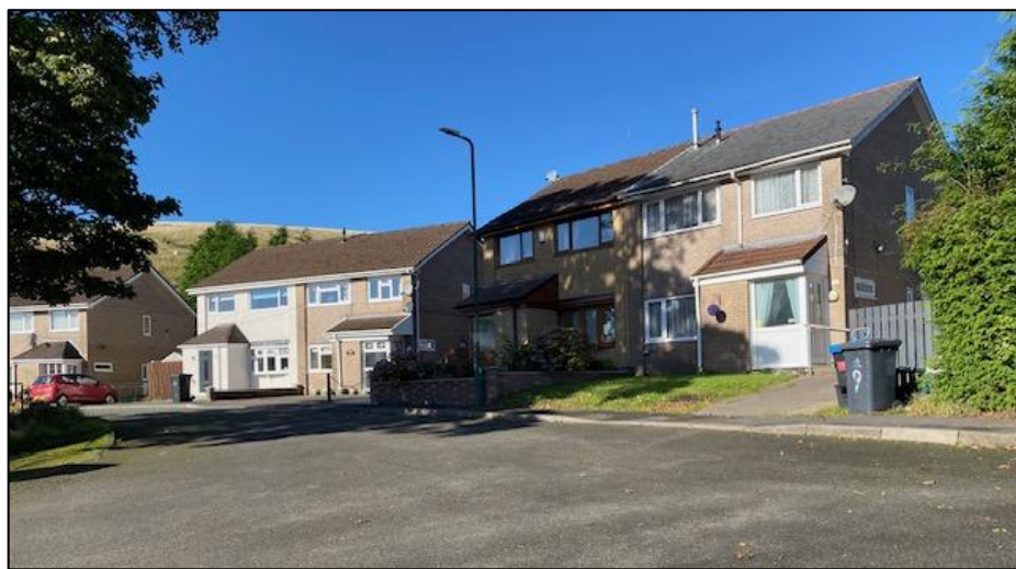
Photograph 6 – Typical House Types at Nearby Oliver Jones Crescent
