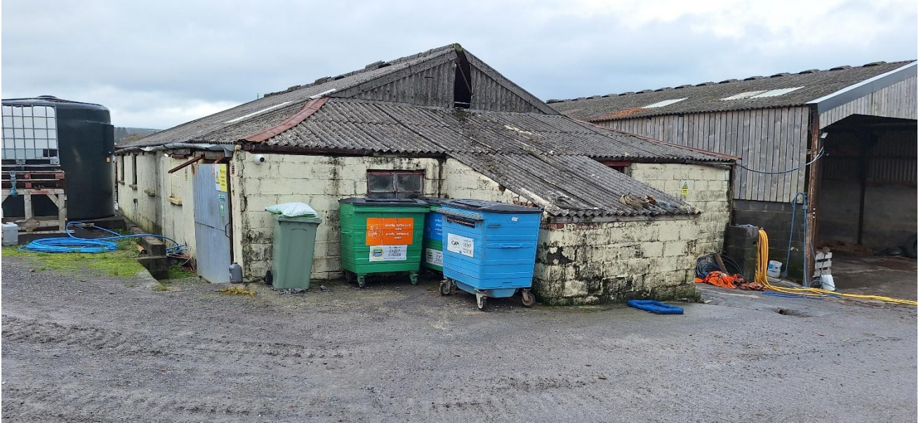
This blockwork shed held no evidence of bats
