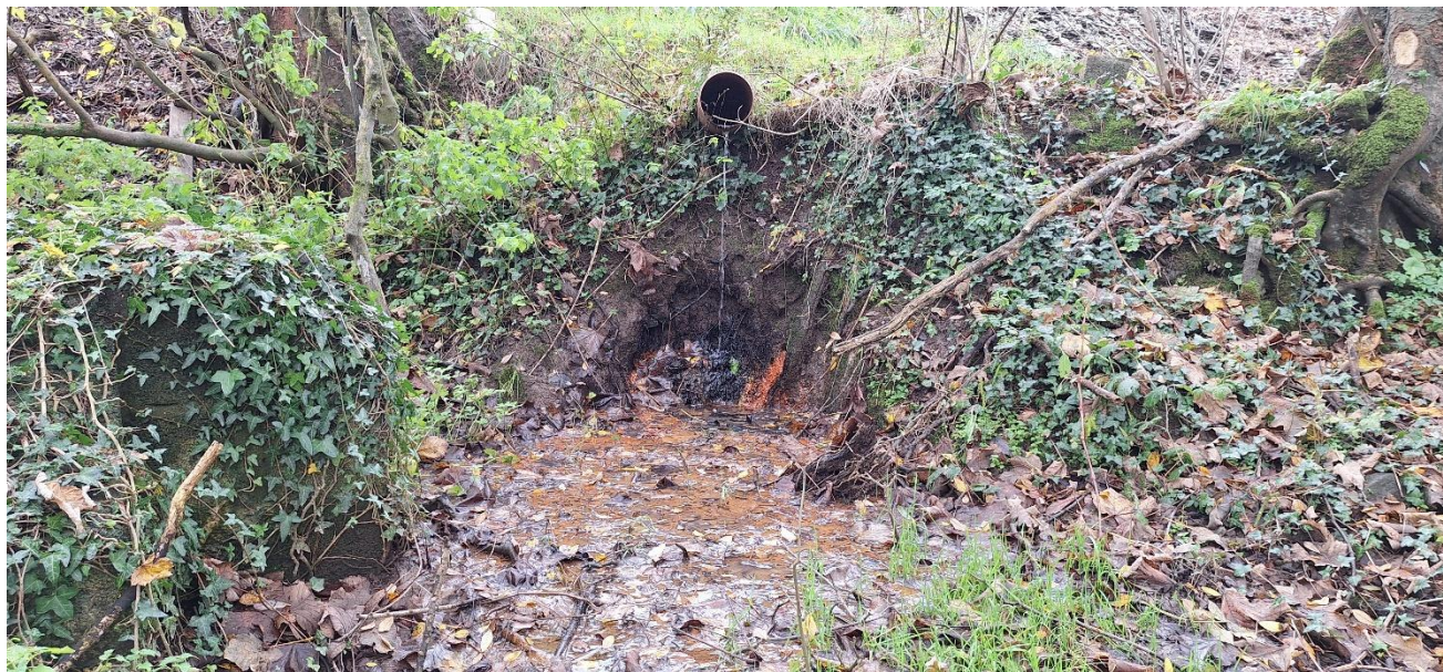
Current outflow from yard towards stream
