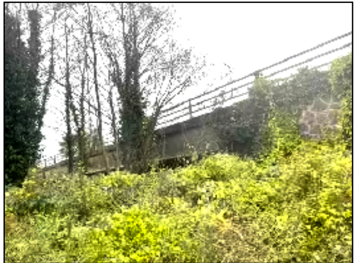
Photo 4. View of far northwest of land adjacent to site. Heilbronn Way road bridge over river.
