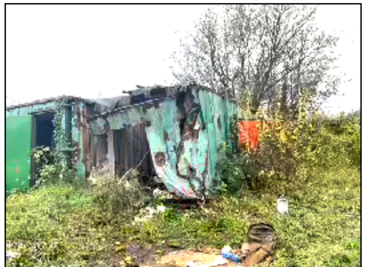
Photo 12. Derelict metal structures in west of site.
