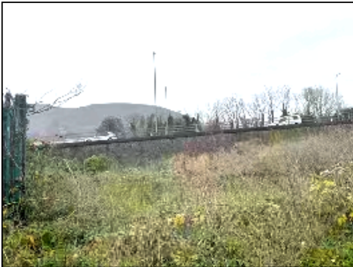
Photo 3. Vegetation within the site and northern boundary wall with Heilbronn Way road.
