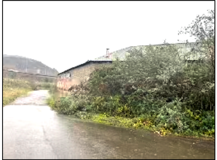
Photo 2. Access road and building along southern boundary of site. View looking east.
