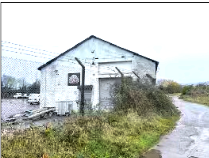
Photo 11. Building bordering south of site.
