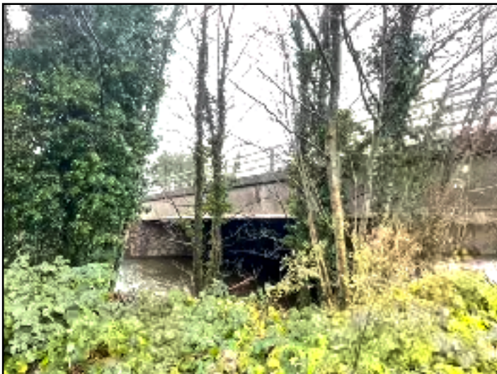
Photo 5. River Afan and Heilbronn Way road bridge.
