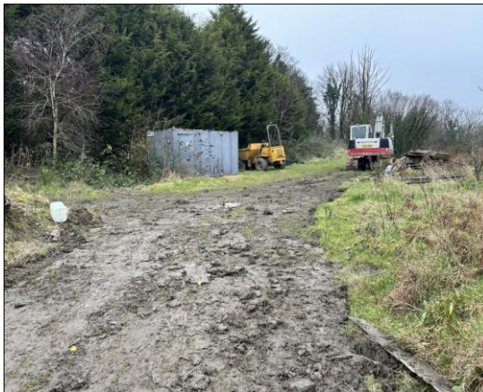
Photograph 4 (View of the Mid-Section of the Site)
