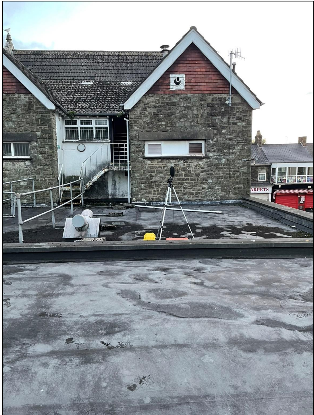
Figure 2 – View of Equipment Location
