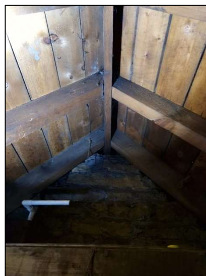
Figure 38 – Tightly Sealed Timber Boards in 2 nd Loft
