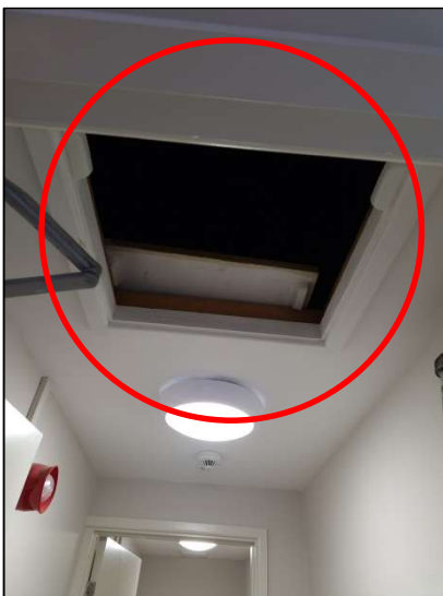
Figure 25 – Access to Void via Hatch in Ground Floor Ceiling
