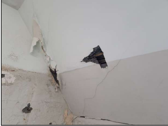
Figure 25 – Access to Void via Hatch in Ground Floor Ceiling
