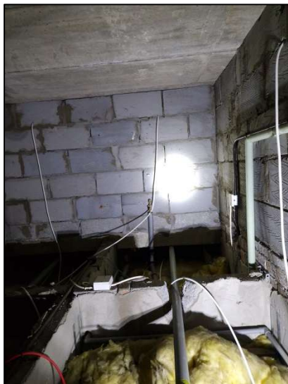
Figure 28 – Interior Details of Void on Ground Floor
