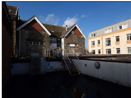
Figure 7 – (NE) Aspect of Main Building as Visible from Flat Roof at Rear of the Building. Looking (W)
