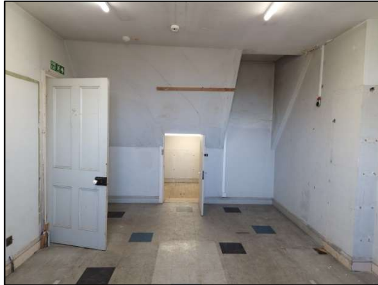
Figure 22 – 2 nd Floor Room with Hatch Permitting Access to Southern Gable, Looking (E)
