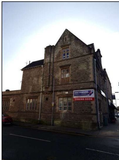
Figure 4 – (N) Aspect of Survey Building, Looking (SE)
