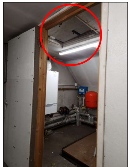
Figure 27 – Access to 2 nd Loft via Hatch in Northern Gable
