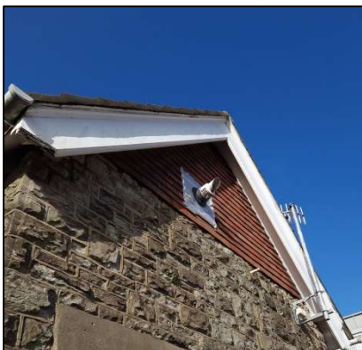
Figure 10 – Hanging Tiles in Good Condition at Apex of Northern Gable at Rear (E) Side of Building
