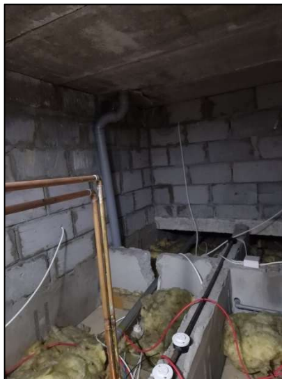
Figure 29 – Interior Details of Void on Ground Floor
