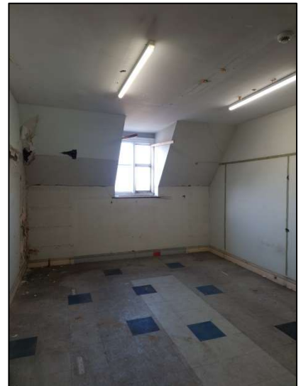
Figure 19 – 2 nd Floor Room and Visible Dormer, Looking (W)
