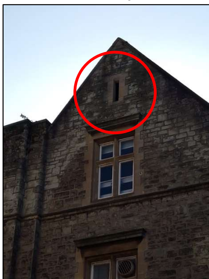
Figure 11 – Slit Window on (N) Wall, which may Permit Access to an Interior Loft Space
