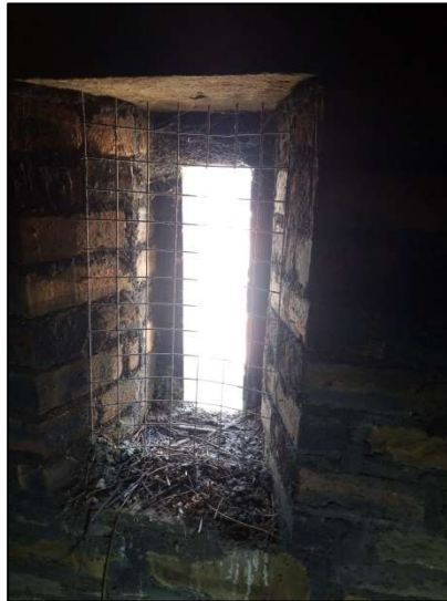
Figure 31 – Arrow Loop Window Detail, with Mesh Covering. Historical Bird Nest can be seen
