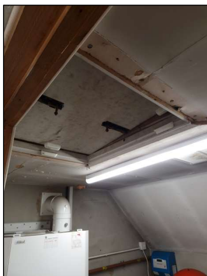
Figure 36 – Access to 2 nd Loft via Hatch in Northern Gable
