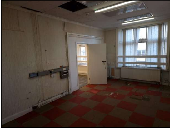
Figure 21 – 1st Floor General Interior, Looking (W)
