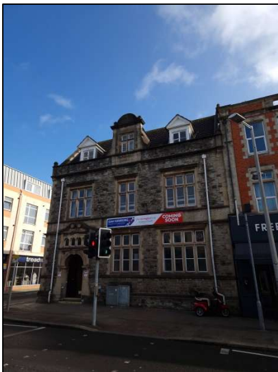
Figure 3 - Front (SW) Aspect of Building with Main Building Entrance Visible to the Left
