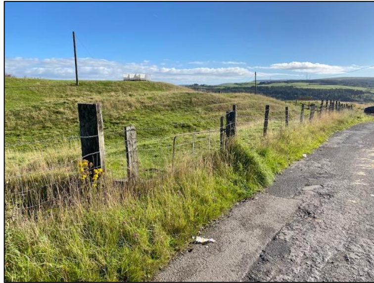
Photo 5 – view along Western Crescent of former tip associated with coal legacy at application site
