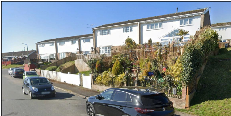
Photo 9 – typical linked, two-storey housing at Cefn Glas
