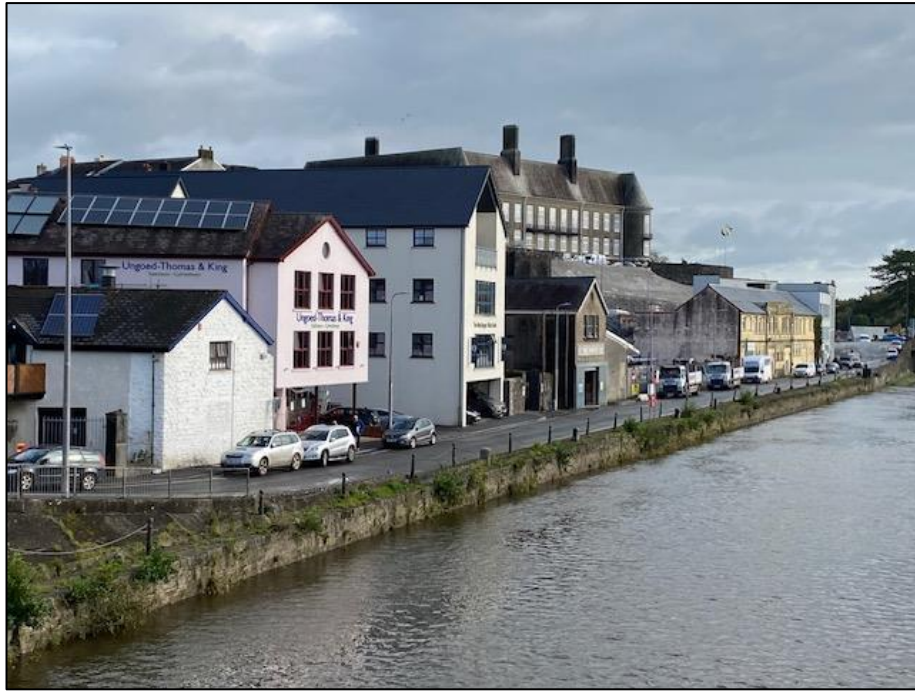
Photo 8 – The whole streetscene of The Quay part of the Conservation Area viewed from King Morgan Bridge
