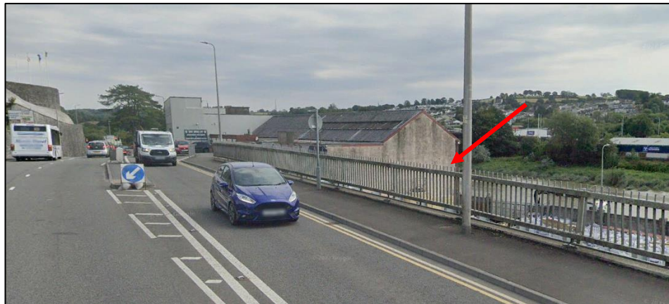
Photo 18 – view from western side of Coracle Way illustrating below highway level of application site
