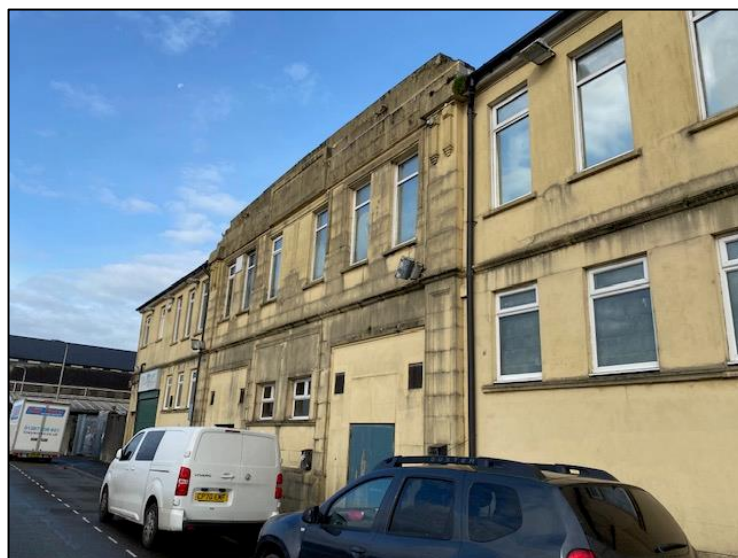
Photo 14 – evidence of white upvc openings upon existing building
