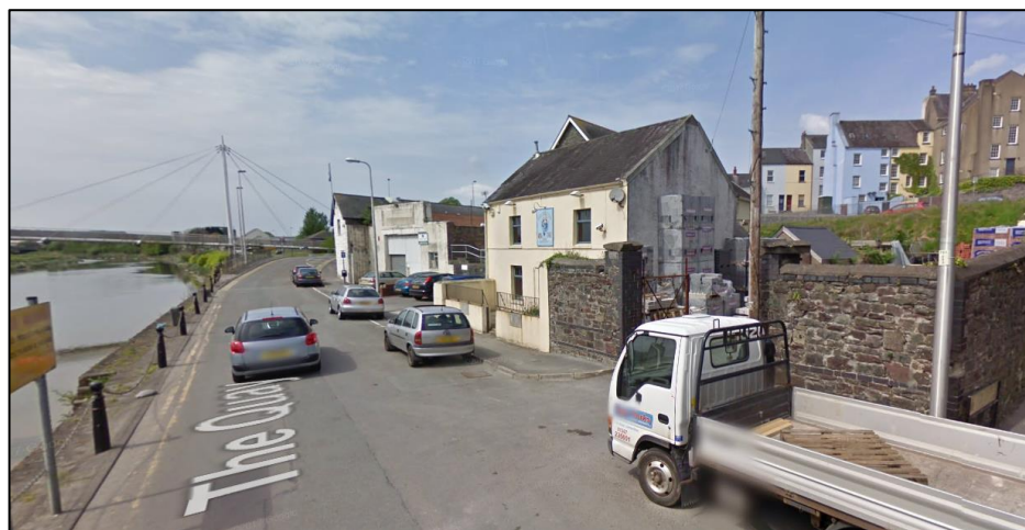
Photo 11 – previous view from same position in streetscene (April 2011) with The Jolly Tar public house and vehicle repair garage in place before demolition
