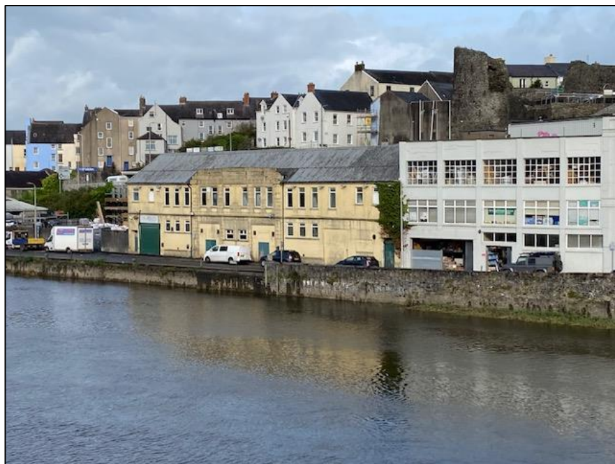
Photo 7 – view of application building, alongside Towy Works, set against the backdrop of Carmarthen Castle and a mix of historic and modern buildings elevated above Coracle Way
