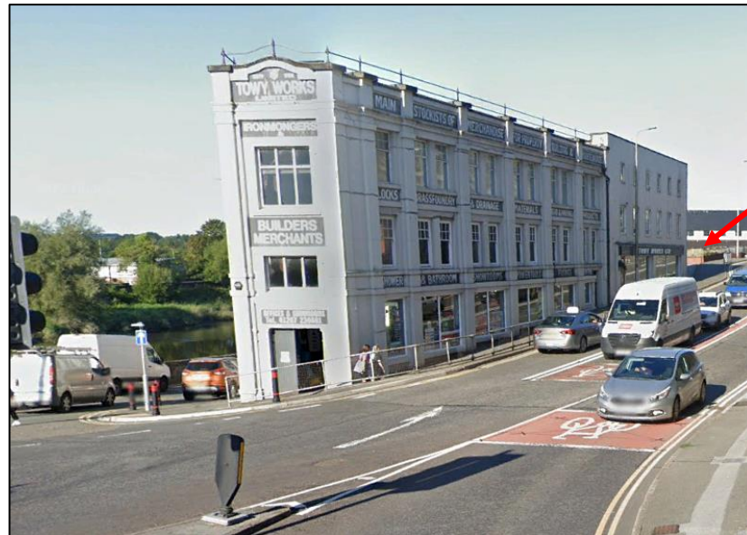
Photo 17 – view of Towy Works from foot of Jail Hill, and recessed position of application building
