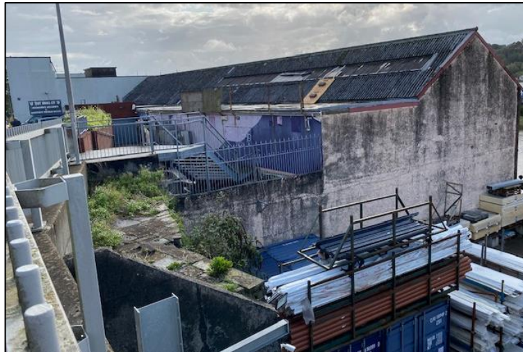
Photo 3 – side elevation to adjoining open yard and range of flat roofed projections to Coracle Way
