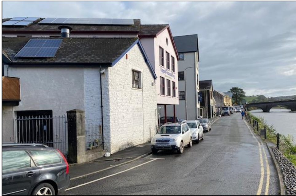
Photo 12 – view from western end of The Quay at expanse of new constructions well in excess of the height of established restaurant (Feb 25)
