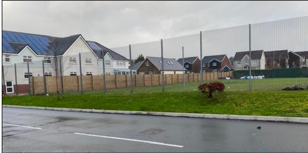
Photo 3 – Application Site as viewed from adjoining retail store car park
