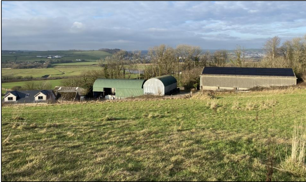
Photo 1 – Agricultural outbuildings at Tyr Mably Farm, located to the north of the application site
