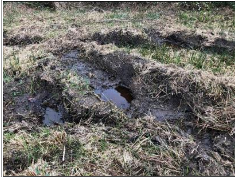
Photograph 6 – Showing Poor Condition of the Site
