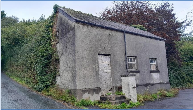
Photograph 5. View of the Building from the southwestern corner.
