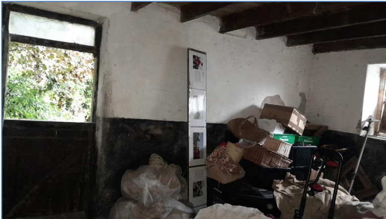
Photograph 15. The internal ground floor space of the Main Building.
