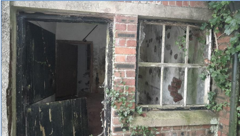
Photograph 19. The internal space of central flat roofed section, with the small western room just visible.
