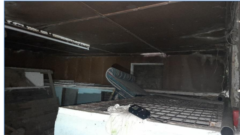
Photograph 16. The ground floor space of the northern section where the ceiling is intact.
