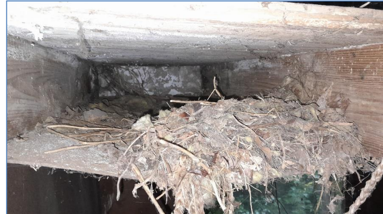
Photograph 20. The exposed ceiling cavity at the north of the Northern Section.
