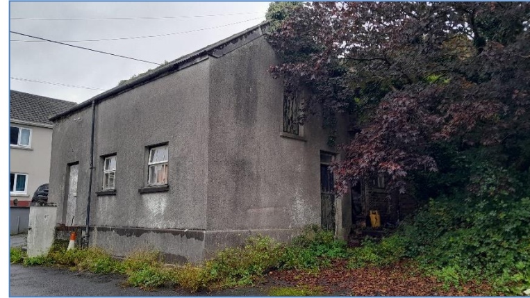
Photograph 6. View of the Building from the southeastern corner.
