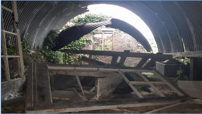
Photograph 17. The upper floor of the northern section (looking south).
