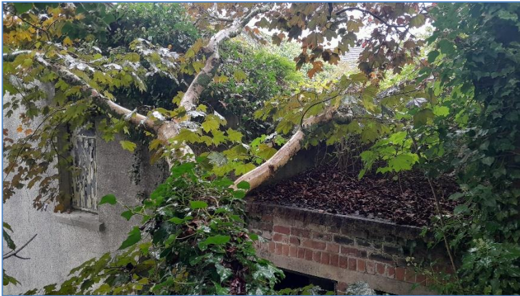
Photograph 7. The flat roofed central section.
