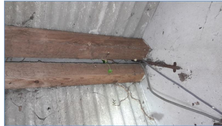
Photograph 14. The double ridge and corrugated fibreboard roof of the main Building.
