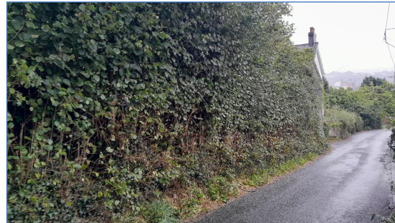
Photograph 12. The western elevation is entirely obscured by the tree line.
