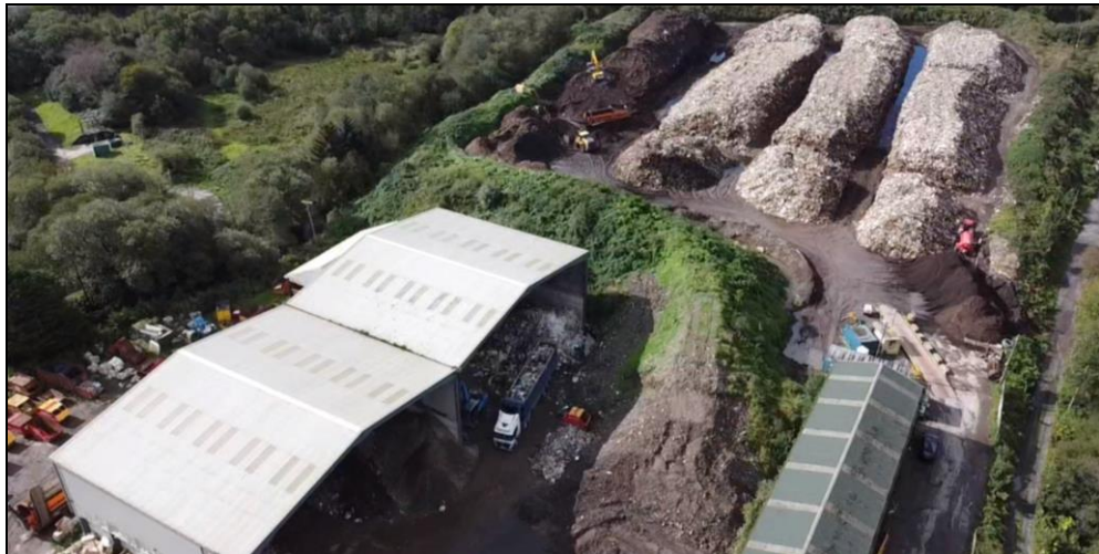
Photo 1 – aerial view over waste wood yard and adjoining MRF sheds and yard
