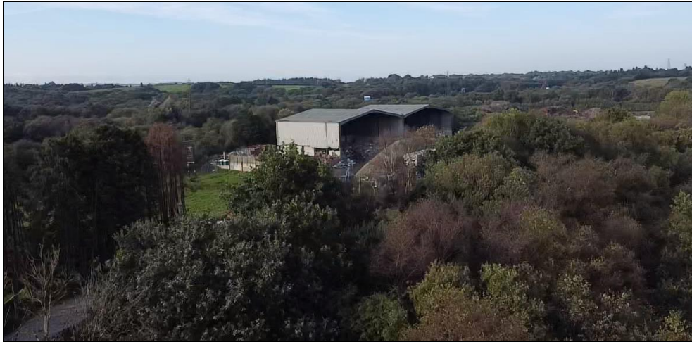
Photo 3 – aerial photo over Bryntywod looking over enveloped railway cutting to site
