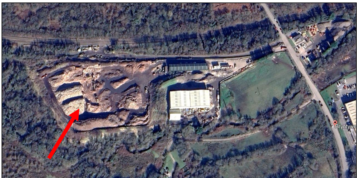
Figure 2 – Google Earth image of the application site locality – July 2024
