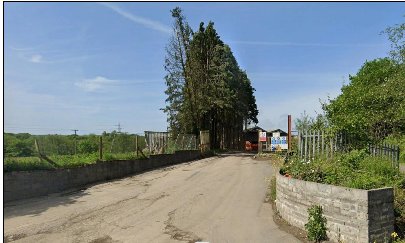
Photo 3 – view from access roadway to existing waste recycling sheds with evergreen tree screen to flank of roadway
