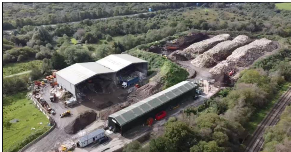
Photo 4 – Aerial view of site waste wood storage and existing waste sorting sheds alongside
