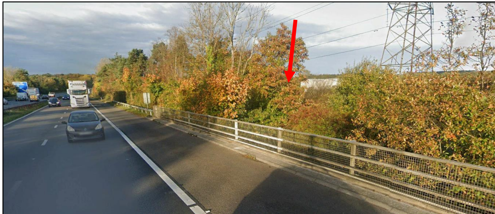
Photo 10 – view from eastbound carriageway of M4 at bridge crossing of Bryntywod
