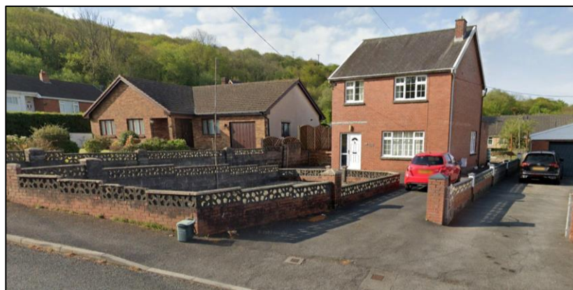
Photo 6 – modern, detached dwellings off Heol Llanelli, opposite site entrance, with heavy brick finish
