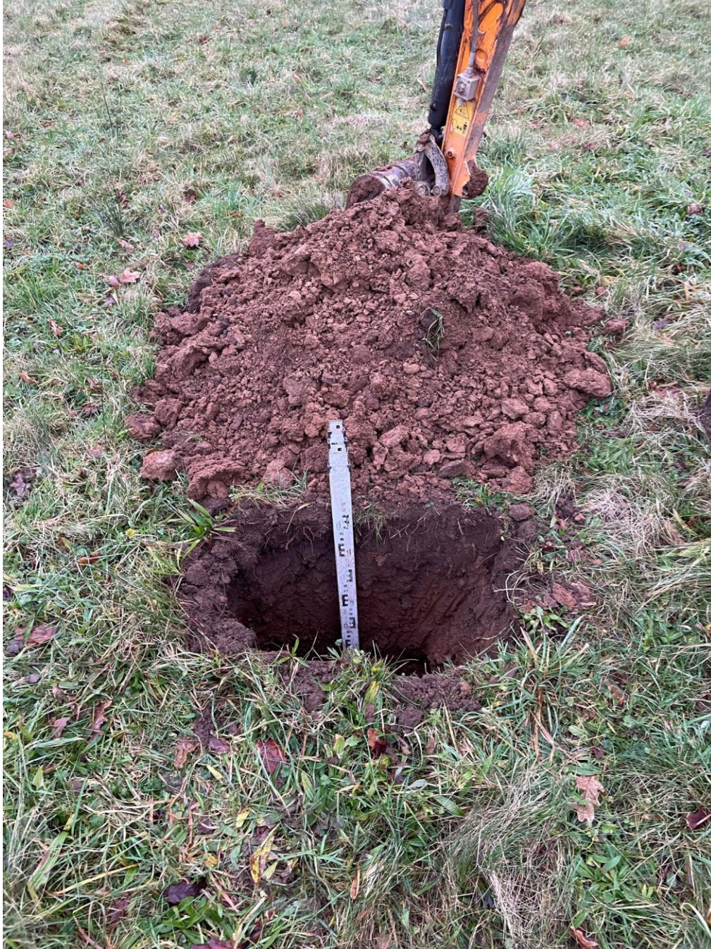
Figure 2 - Test pit 1 during excavation
