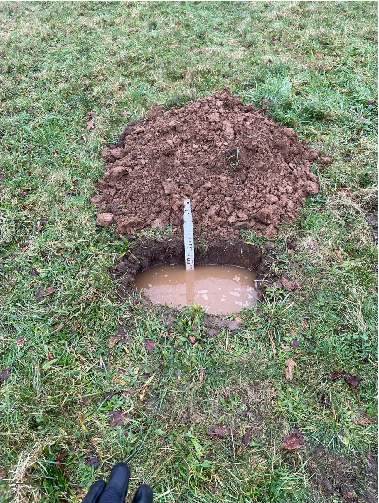
Figure 3 - Test pit 2 after filling
