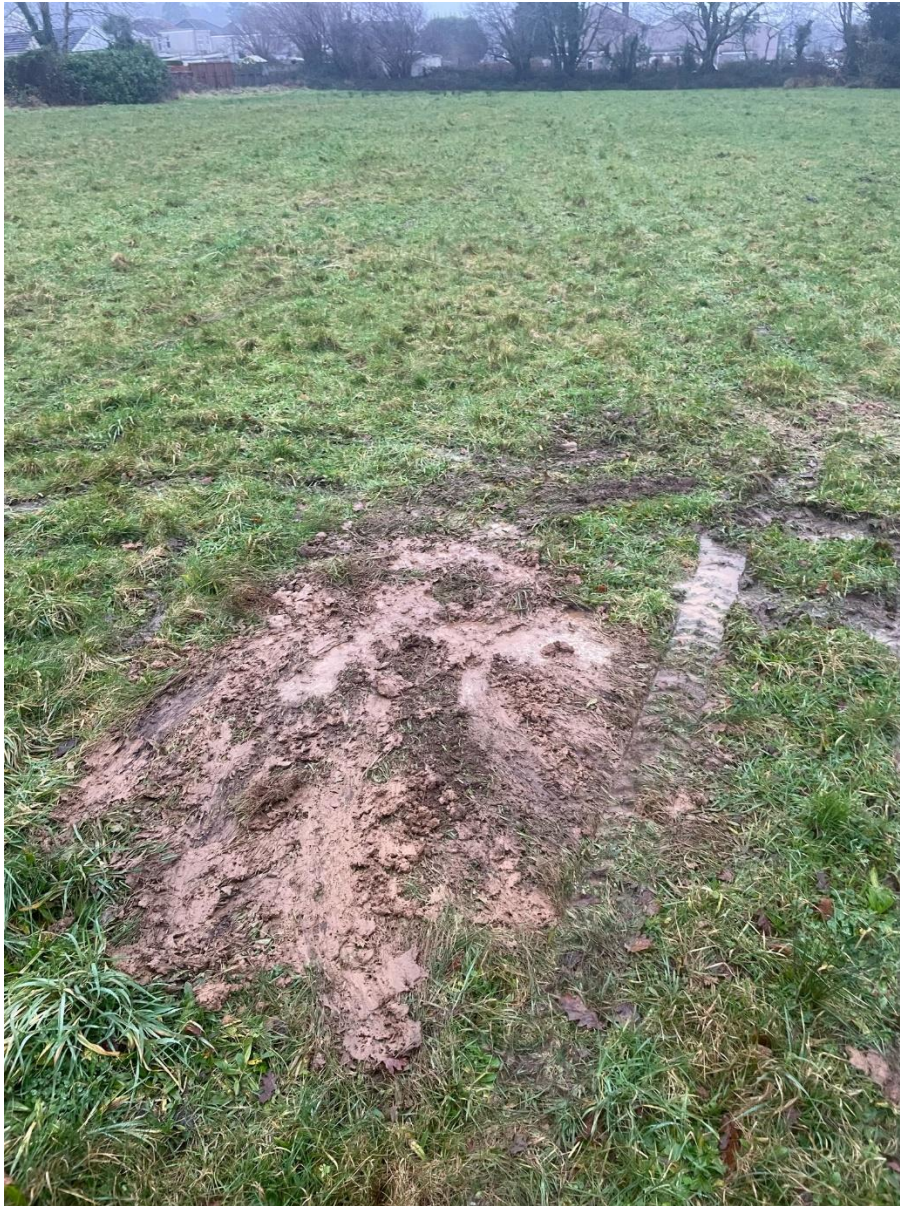
Figure 6 - Test pit remediation
