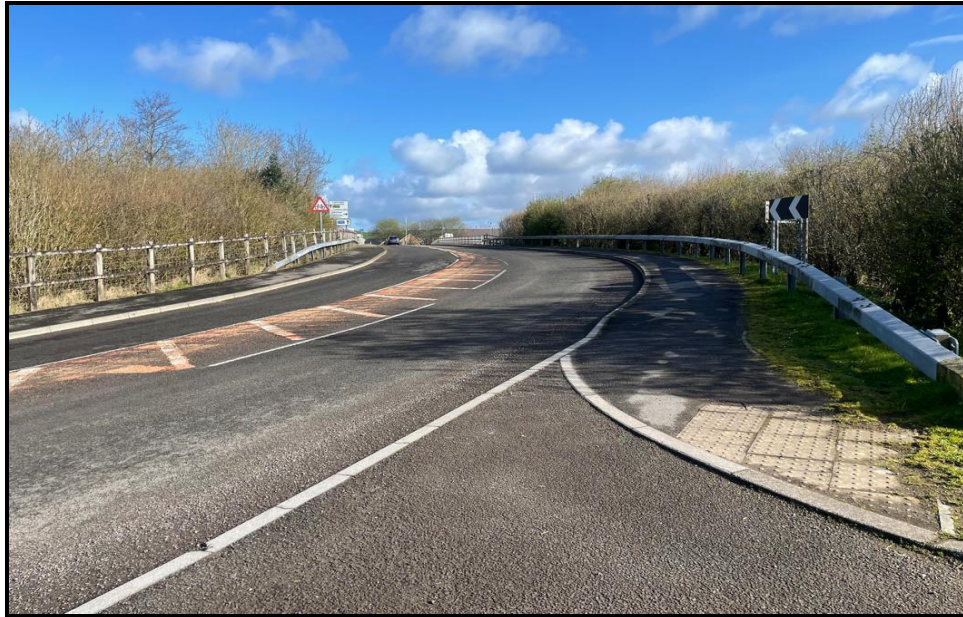
Photograph 3 – The Visibility Splay Facing North from the Site onto St Clears Road
