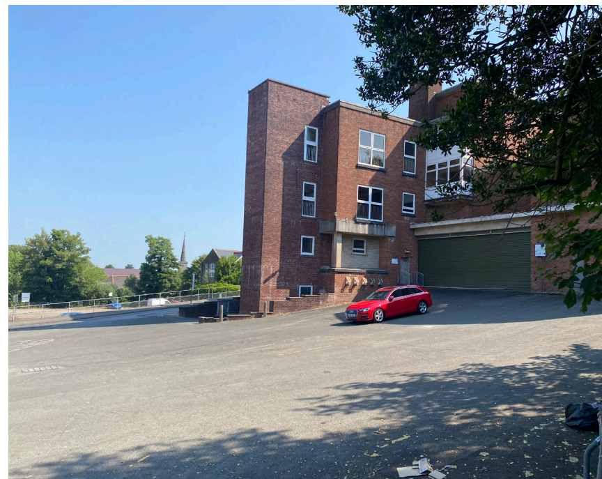
Rear of former library - slope of land is clearly evident
