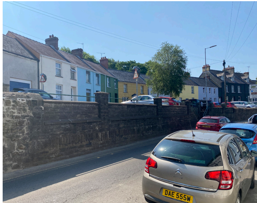
Retaining stone wall and rendered terraces along Dew Street
