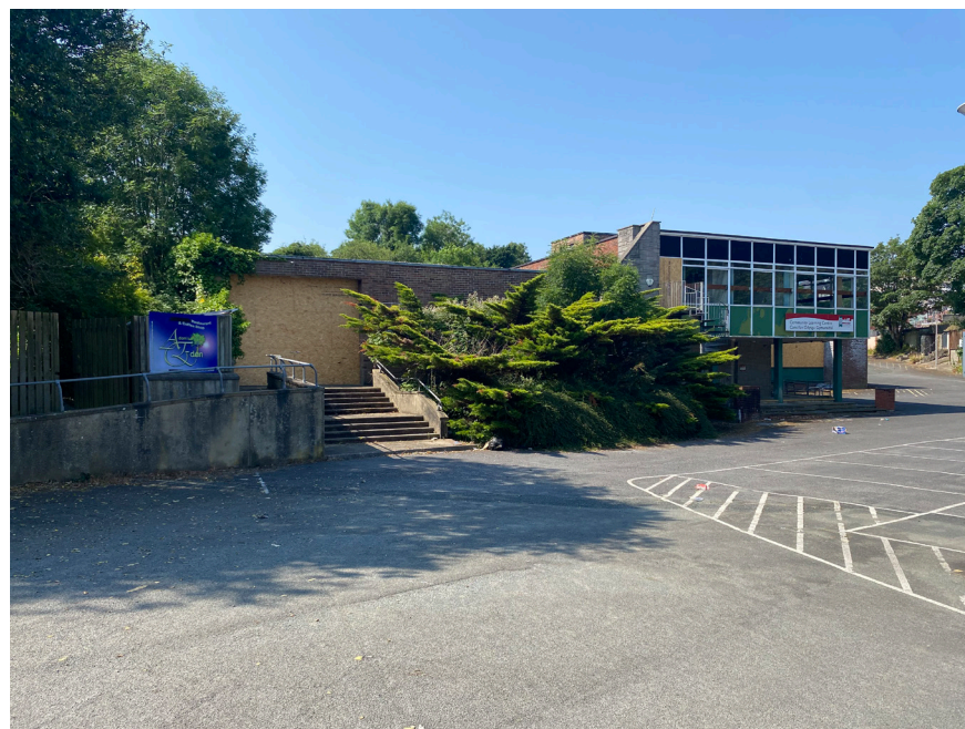
Former education building, path to rear of Dew street properties to left
