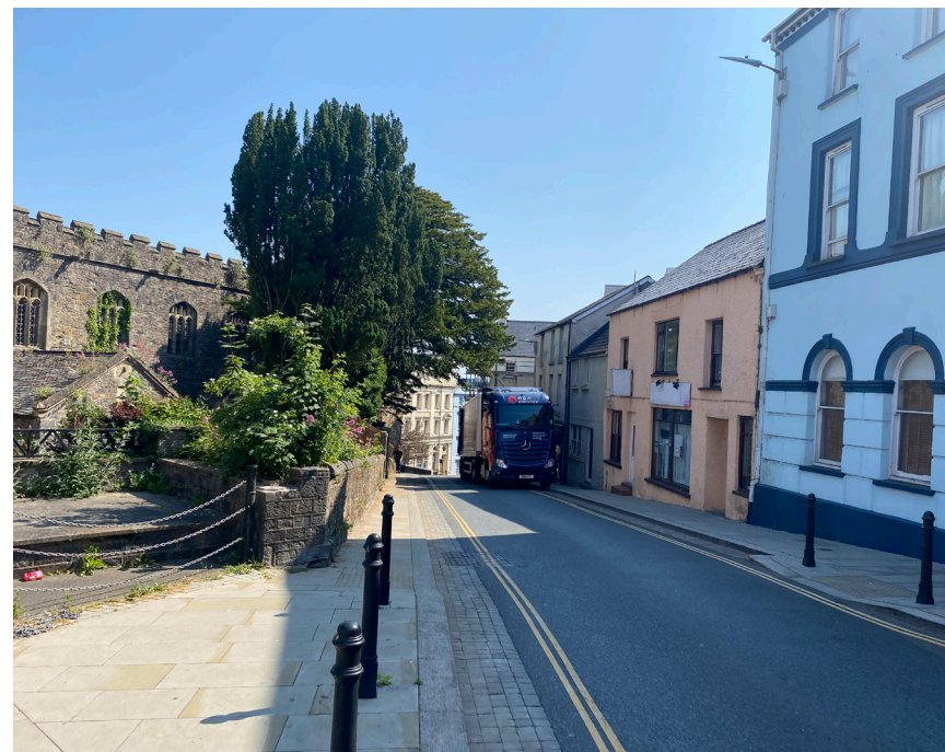
St Mary's Church left, and render facades along High Street
