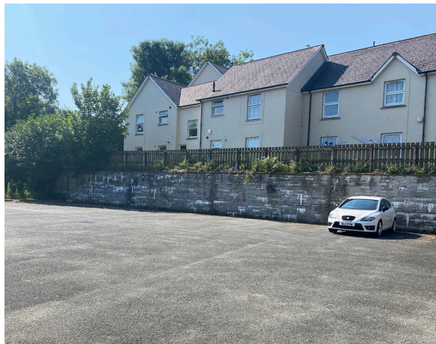
South-West boundary - retaining wall to Barn Court
