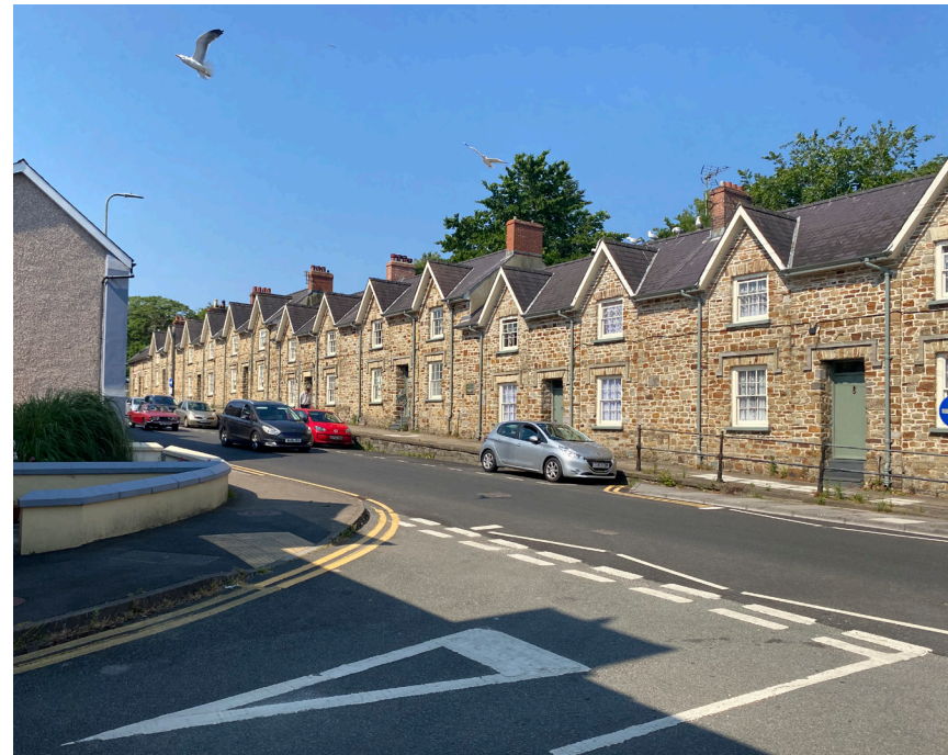
Stone terraces (listed) along Barn Street
