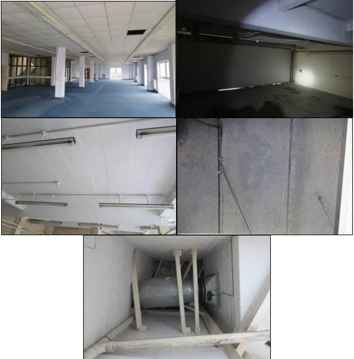
Additional interior images showing the absence of any bats or their signs.
