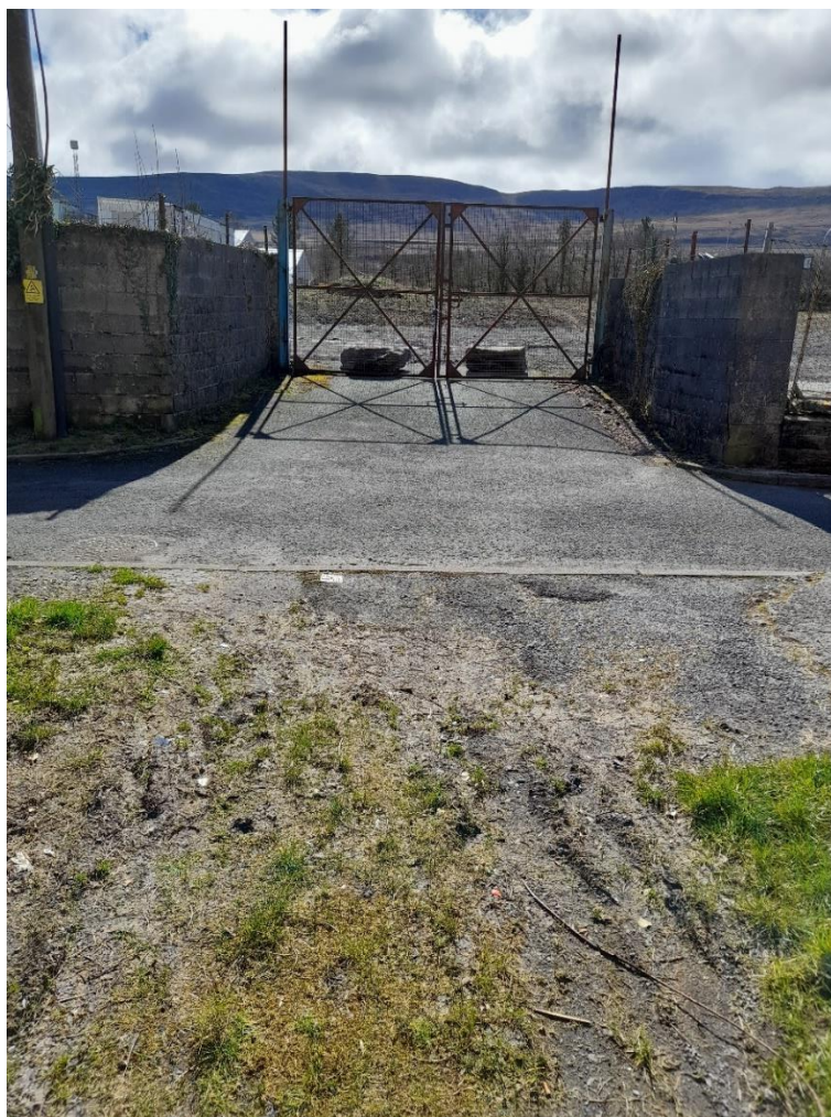
Plate 2: Existing gated site access
