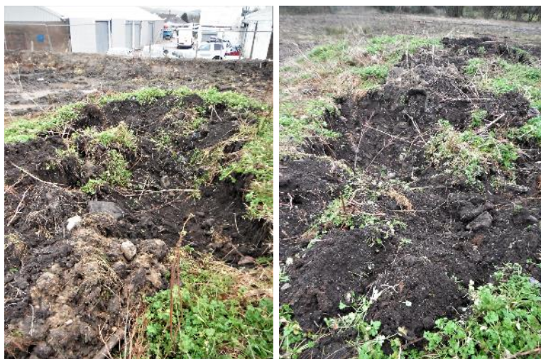
Plate 17: Areas of excavation on the tops of the vegetated mounds (Target notes 3&4)
