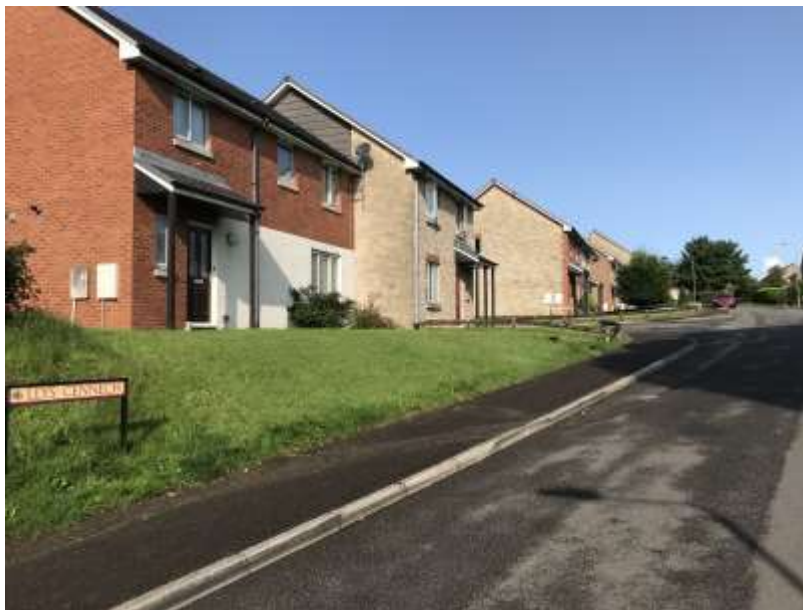
Photo 6 – extent of Parc Morlais junction opposite frontage field with modern residential properties
